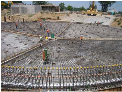
Waste Water Plant, St. Louis Client: Tarlton Corp
